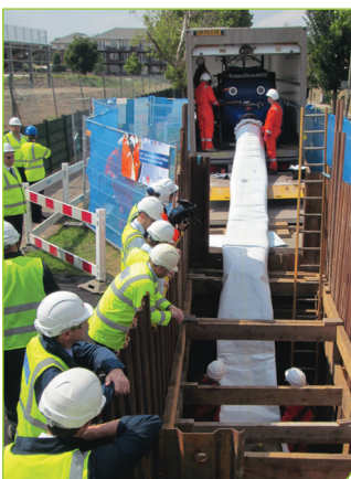
The CIPP technique being monitored by engineers.
