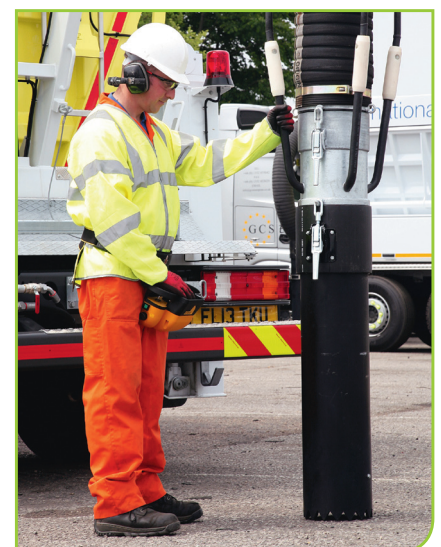
The Core and Vac process taking place.
